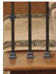
Open Tread Bottom Connection
